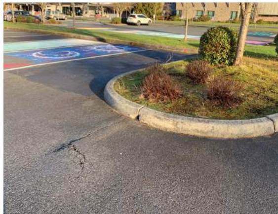
▲ Cracks in asphalt, presumably due to root growth.
