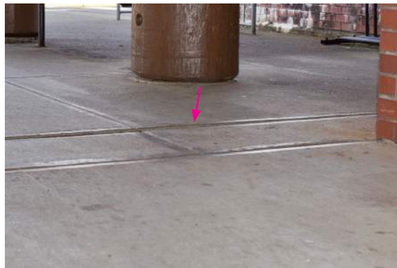
▲ Raised lip in concrete paving at main entry.
