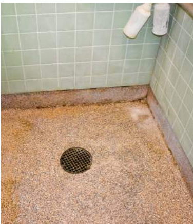
▲ Cracking at floor-to-wall seam in acrylic resin flooring.
