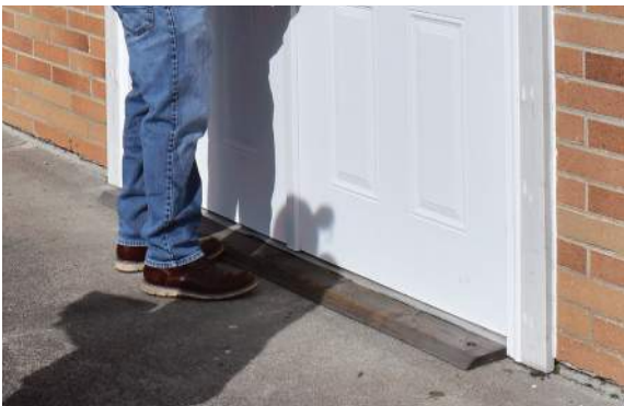
▲ Modify exterior door threshold to allow for equipment to wheel in & out of space.
