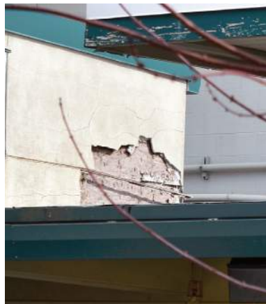
▲ Large area of stucco is missing on south wall.
