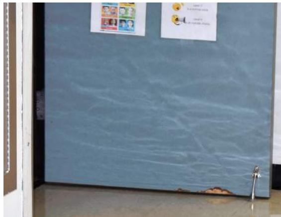
▲ Plastic laminate facing at interior door is beginning to show signs of age.
