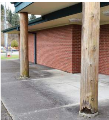
▲ Degradation visible at wood peeler pole columns.
