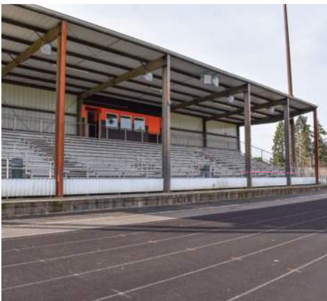
▲ Middle school grandstand. Dashed line showing location of missing guardrail. ▲ Missing section of guardrail at middle school grandstand.
