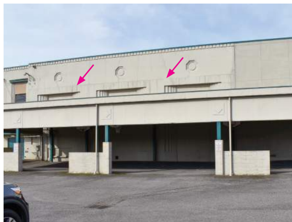
▲ Significant cracking in stucco at south side of the gymnasium.
