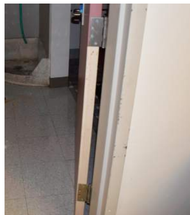
▲ The plastic laminate finish is peeling away from the interior doors.
