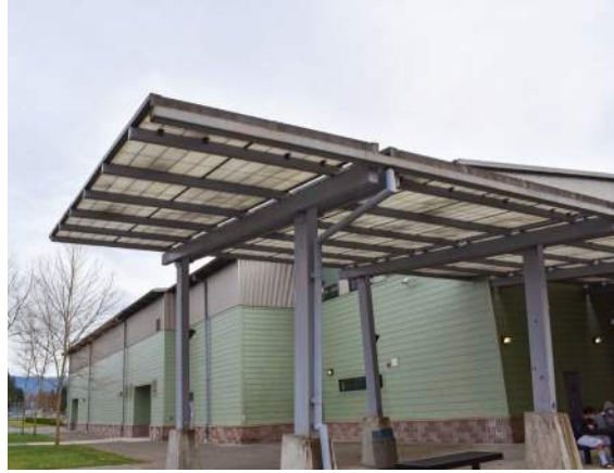
▲ Debris build up on rear translucent panel canopy.
