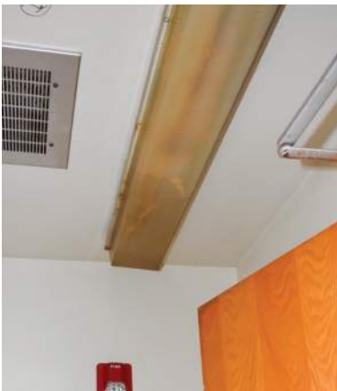
▲ Standing water in the light fixture at the staff restroom.
