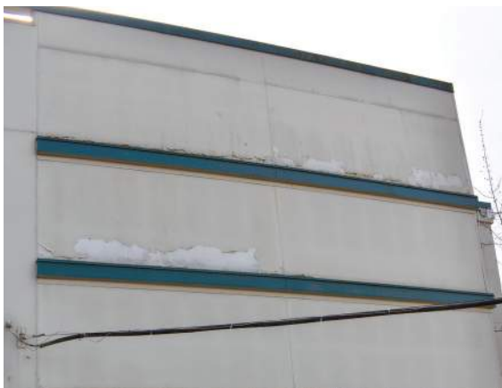
▲ Damage to fiber cement panels at the Crossroads / Administration building.
