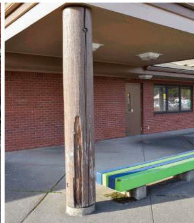
▲ Checking and rot apparent at multiple peeler pole locations.
