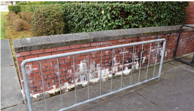
▲ Efflorescence at entry wall
