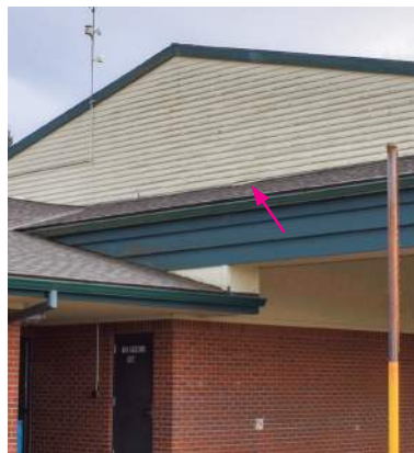
▲ High wall over the covered play area showing weathering at cedar siding and slipped piece of through-wall flashing.
