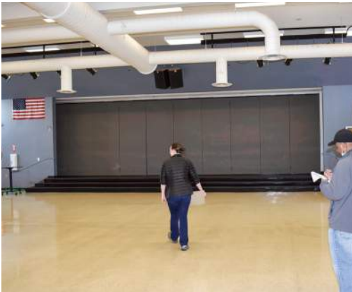
▲ Stage operable partition is no longer functional.
