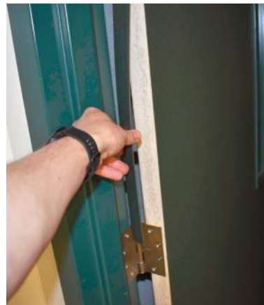
▲ De-laminating interior door.
