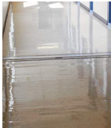
▲ Missing VCT at second floor expansion joint.
