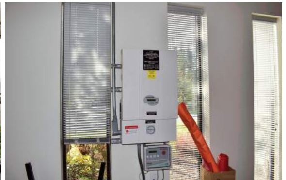
▲ The inverter for the PV array above the A-wing classrooms is located in the satellite workroom on the first floor.
