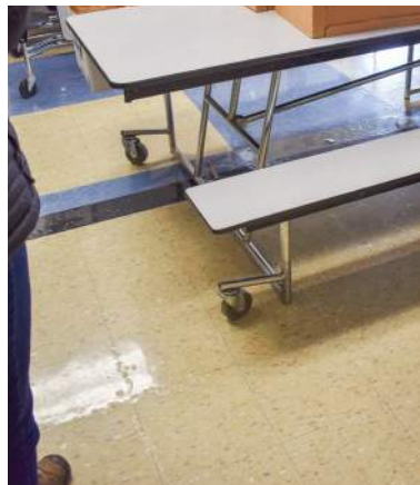
▲ Bubbling in VCT at Multipurpose Building.
