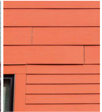
▲ Butt joints at fiber cement siding should be periodically re-caulked.
