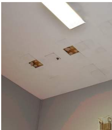
▲ Acoustical tile detaching and falling from gym ceiling.
