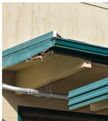
▲ Deterioration at the fascia.
