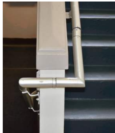
▲ Re-align and secure elements of handrail at administration stair.
