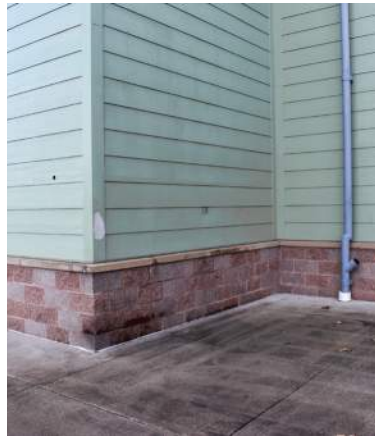
▲ Small holes in fiber cement siding.
