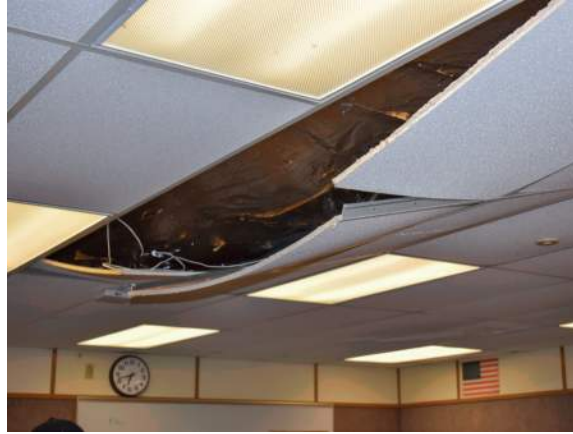
▲ Broken ceiling support system at Portable P4.
