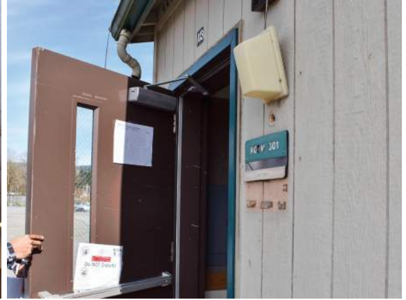
▲ Secure exterior light fixture at Portable P4.
