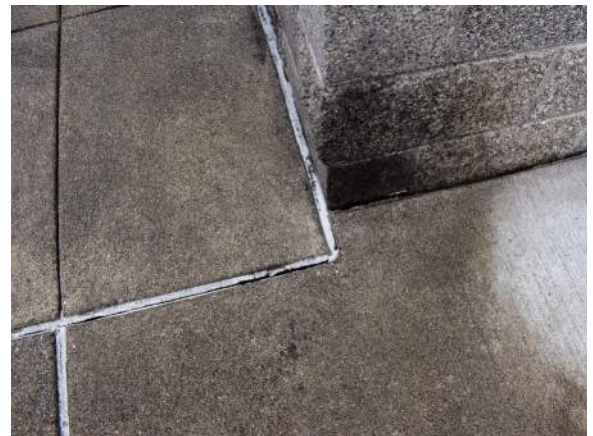
▲ Sealant has deteriorated, or is missing at expansion joints along the face of building and across the plaza.
