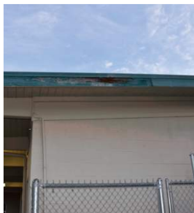
▲ Deterioration at the fascia.
