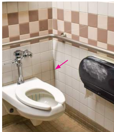
▲ Tile is cracking at corner seams.
