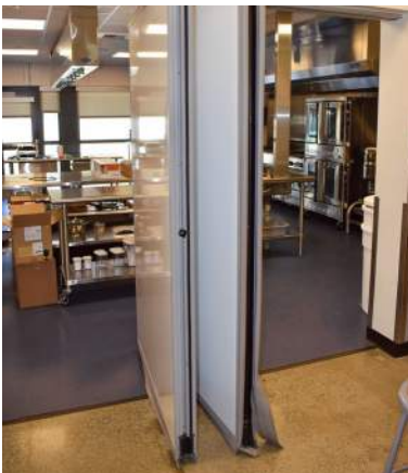
▲ Slipped seals at operable partitions in STEAM building.
