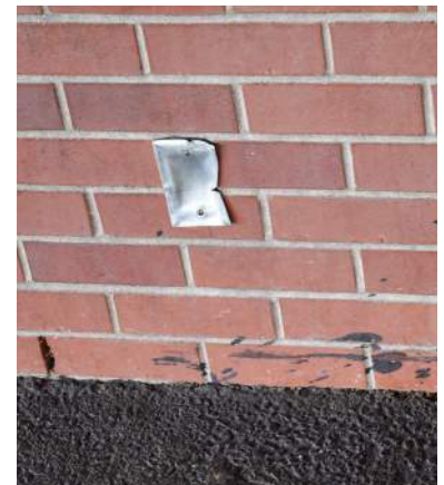
A Damaged junction box cover at attached covered play area.
