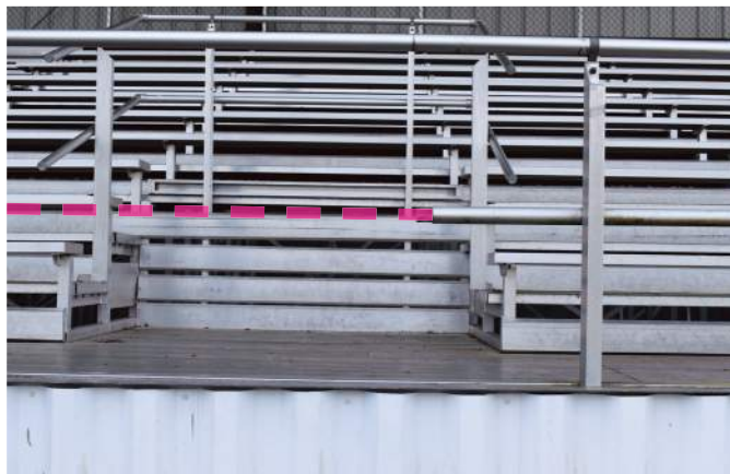
▲ Middle school grandstand. Dashed line showing location of missing guardrail. ▲ Missing section of guardrail at middle school grandstand.
