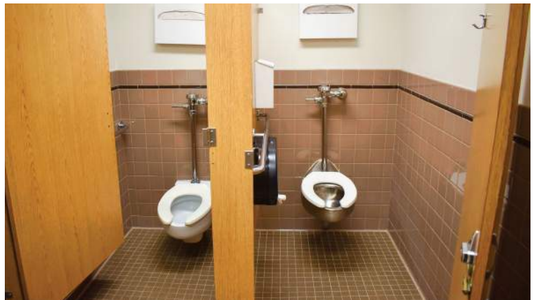
▲ Restroom does not appear to meet accessibility standards with regards to floor clearances and grab bar installation.
