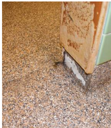
▲ Cracking in flooring, and wainscot water damage.
