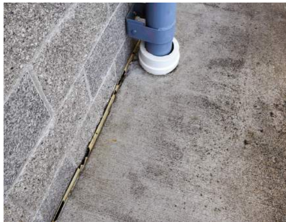
▲ Sealant has deteriorated, or is missing at expansion joints along the face of building.
