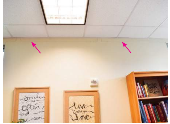
▲ Crack at exterior wall of Classroom B219.
