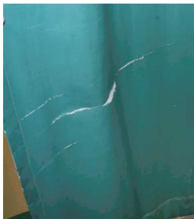
▲ Wear and rips in the operable divider curtain at the gymnasium
