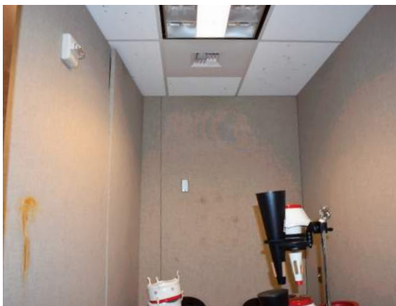
▲ Damage at ceiling and acoustical wall panels in practice room.
