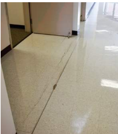
▲ Pronounced cracking in VCT at corridor.
