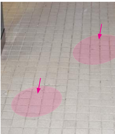
▲ Depressions in ceramic floor tile at restroom.
