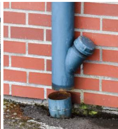
▲ Secure sleeve to base of downspouts.
