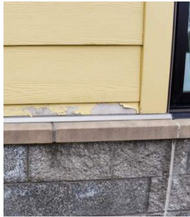
▲ Peeling paint at fiber cement siding indicates moisture intrusion at fiber cement termination.
