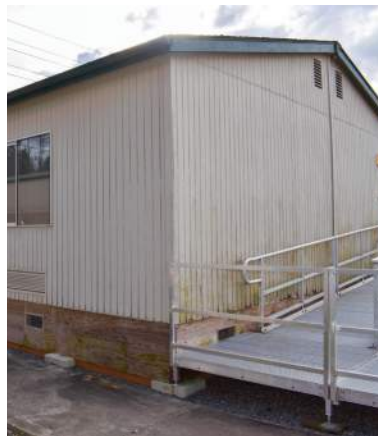
▲ Visible weathering of the siding at Portable P5
