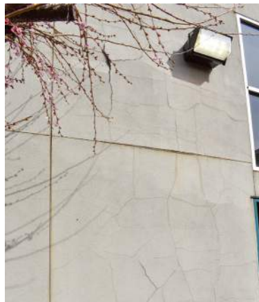
▲ Visible cracking in stucco siding at south wall.
