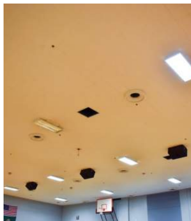
▲ Missing HVAC grilles and broken lighting at gym.
