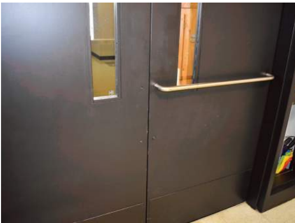
▲ Missing door hardware at entry door.
