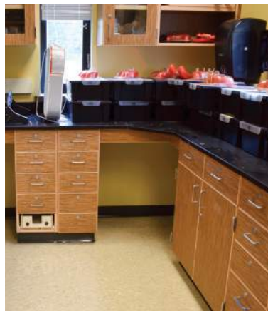
▲ Science casework with missing drawer fronts and drawer hardware.
