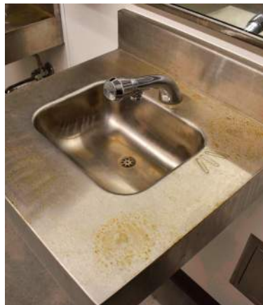
▲ Firework damage to turf field at Tiger Stadium. ▲ Surface rust at stainless steel sinks. ▲ Cracking at tennis courts.
