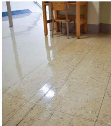
▲ Cracking in VCT at second floor.
