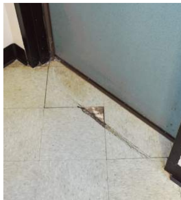
▲ VCT damage at mechanical room entry door.
